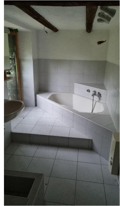
Bad EG Scheune
